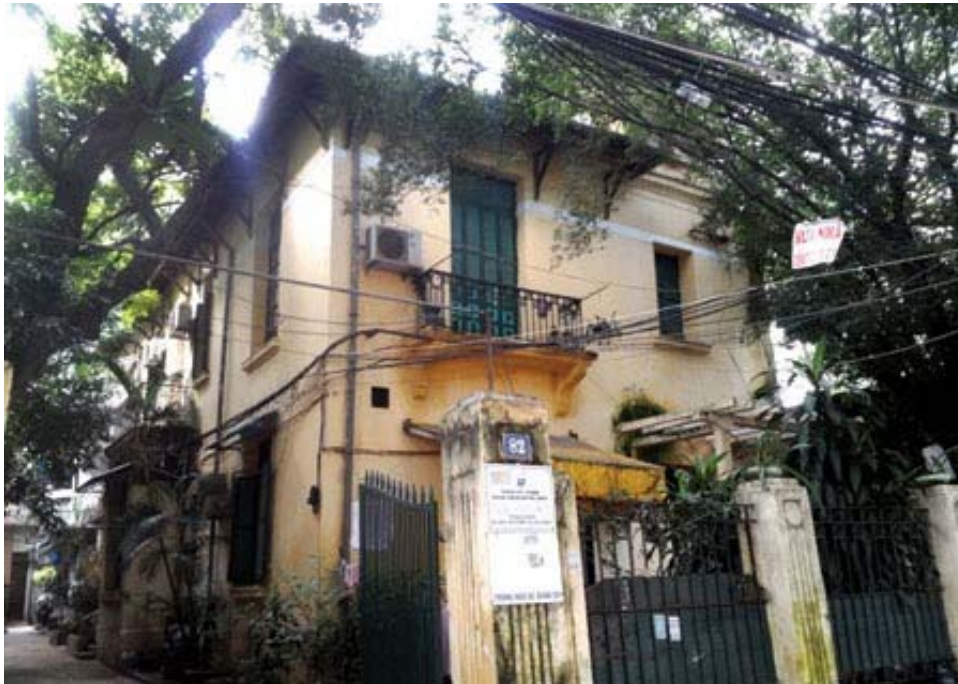
Downtrodden: A French-style villa in Quan Su Street that is home to 10 households. — VNS Photos Doan Tung
